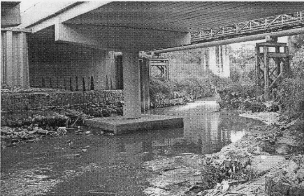
Figure 5 : Plentong River Bridge (flow from top right to bottom left)
